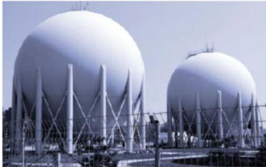
Spherical tanks are often used to store oil and gas at refineries, since this shape is the most economical to build.
